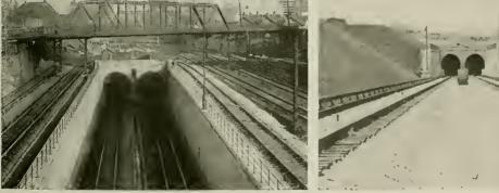
CANADIAN ENTRANCE TO TUBE THE AMERICAN ENTRANCE TO TUBE This railroad tube under the Detroit River Is 2.6 miles In length, including its approaches. It consists of two steel and concrete tubes 21% feet in diameter. The Detroit approach is the Michigan Central Station
