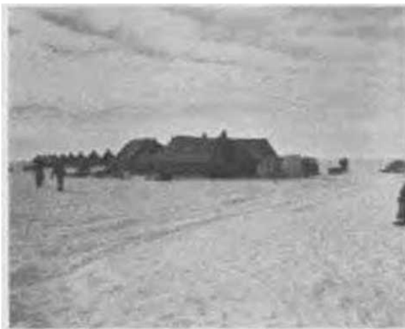
Figure 188. View of mess tents from the southwest.
