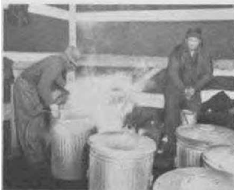
Figure 48. Inside snow melting shelter. Behind steam is Aeroil No. 98 Steam Thawing Unit. Man on left is holding steam pipe in G. I. can partly full of snow; man on right is pumping air into tank for burner which is bottom of steam thawing unit.
