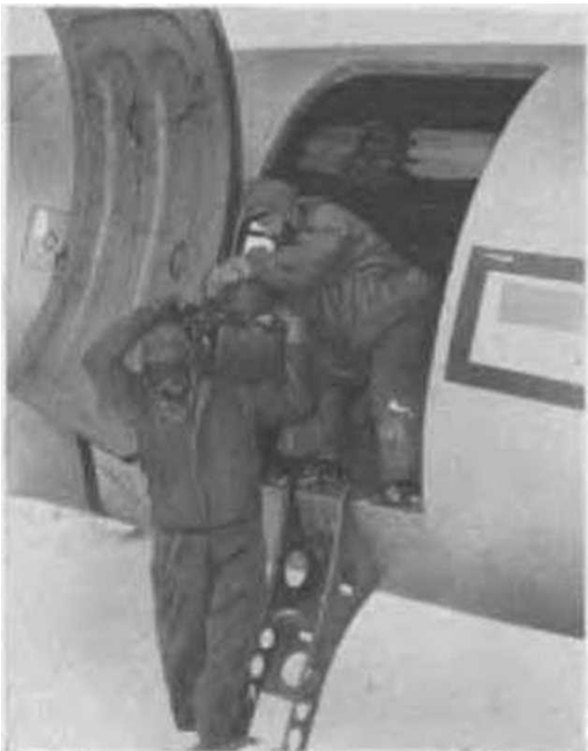
Figure 250. Installing trimetrogon cameras in R4D.
