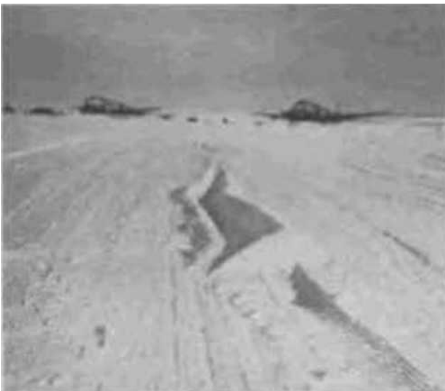
Figure 65. R4D (C-47) tracks on ski runway No. 1 which show that it was not evenly compacted.
