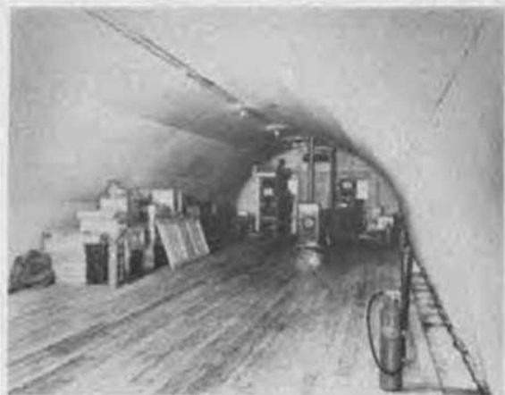
Figure 46. Inside of Quonset hut at Little America III. Note gap in floor on right side so that warm air can circulate to the left and come up through cracks in center of floor (cracks not visible).
