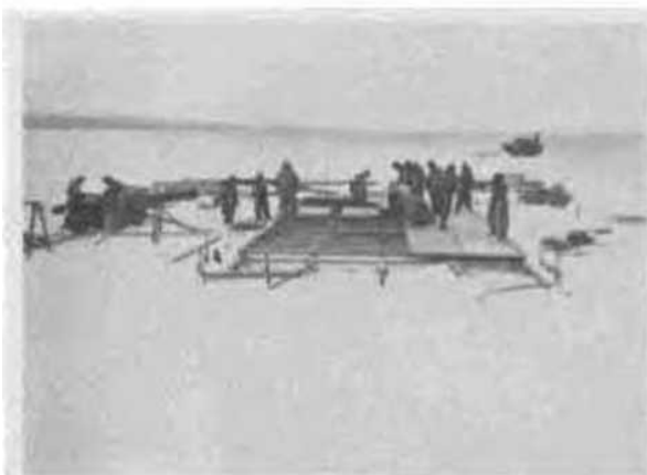
Figure 42. Floor frame assembly for Quonset hut. Note near left corner metal sills are resting on 4-by 4-inch members, which are resting on 2-by 10-inch pieces, which are resting on and perpendicular to floating dunnage foundation.
