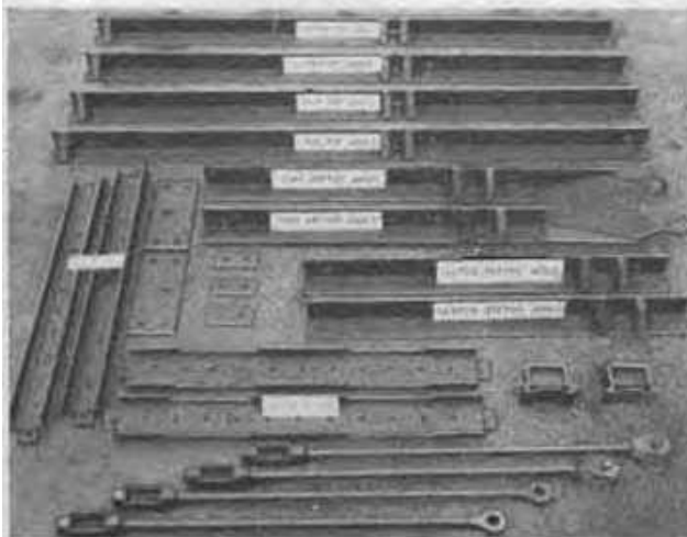
Figure 13. Package shot (disassembled) pontoon snow drag.
