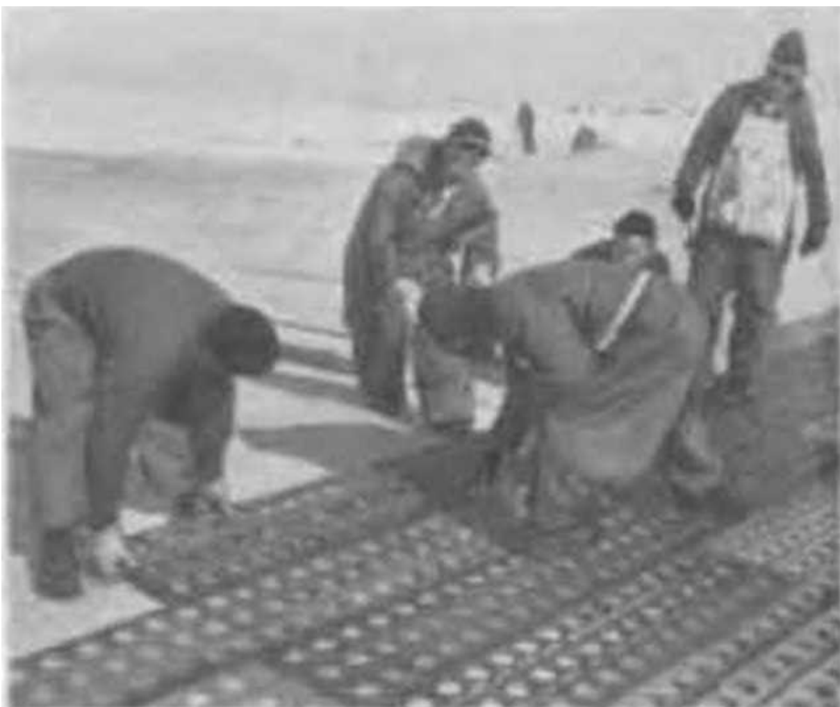
Figure 51. Laying PSP on burlap which was laid on undisturbed snow.
