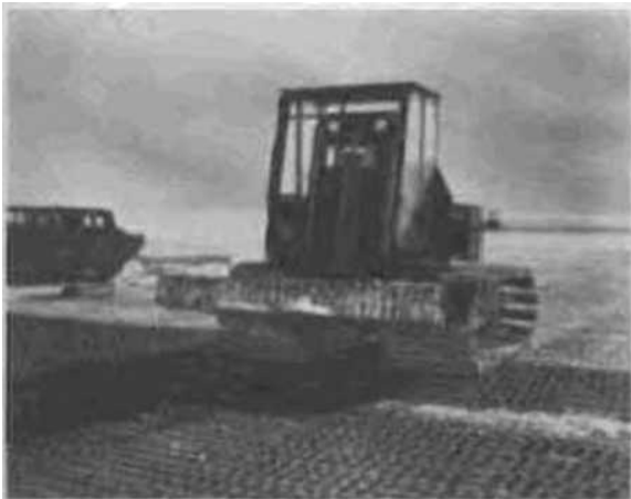
Figure 95. Fingerlift distributing pierced plank on the airfield.
