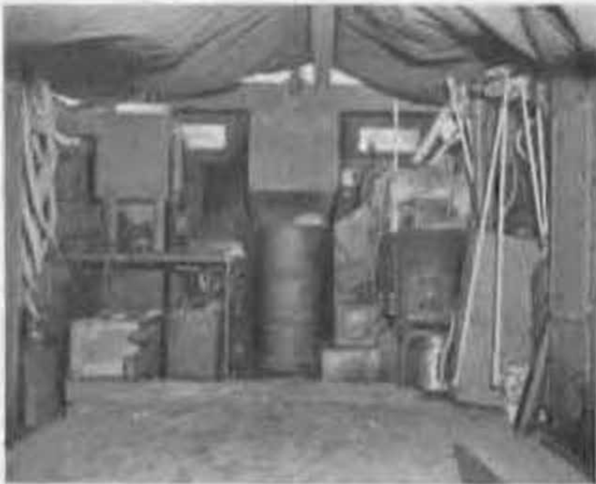
Figure 238. Radio and interior installations in LVT-4.
