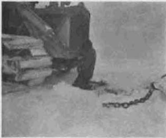
Figure 113. Attaching towing bridle of Go-devil sled to front of tractor.
