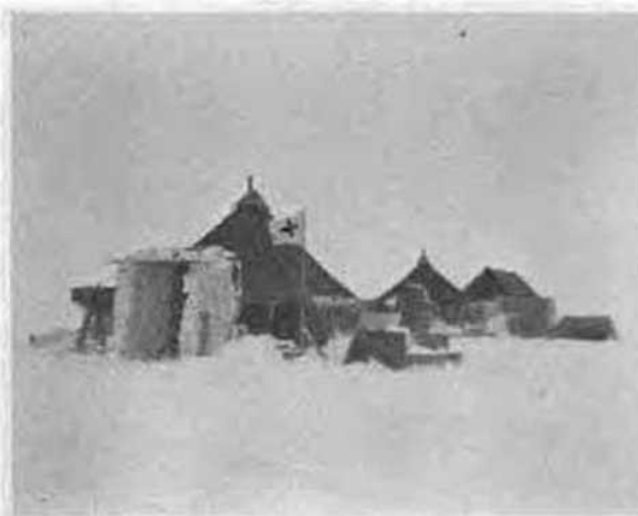
Figure 185. Hospital tent, showing entrance formed by snow blocks to break the wind. Plywood door on inside completes this entrance.
