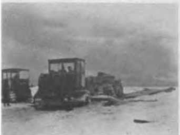
Figure 19. Bridge crossing crack in bay ice (PSP was put on top of one of the two bridges as wearing surface).
