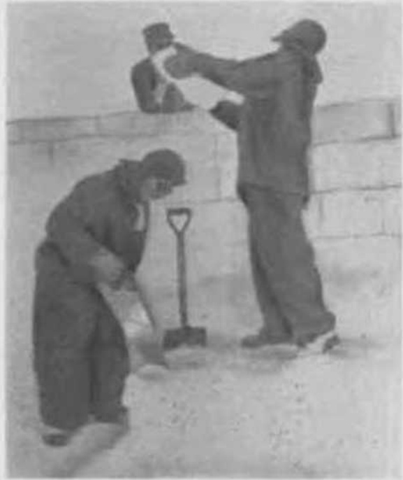
Figure 37. Digging hole for frozen food storage. Note snow being sawed into blocks for easier handling.
