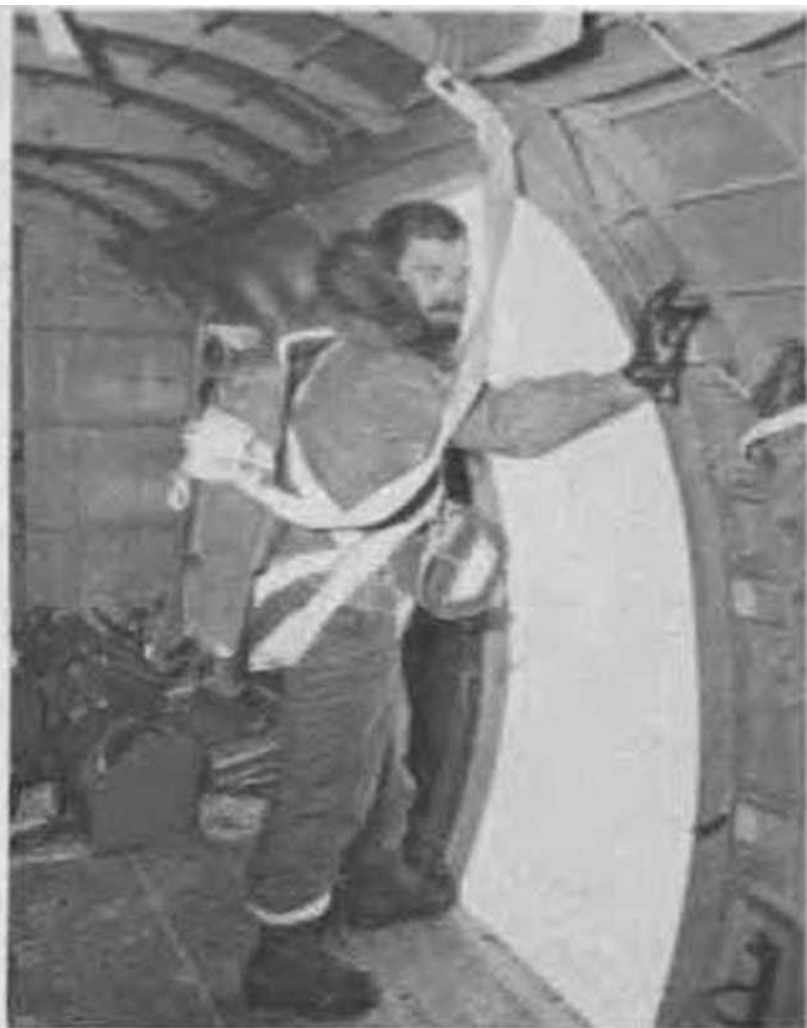
Figure 163. Sgt. S. A. London just prior to making parachute test jump. Note T/5 parachute assembly and static line.
