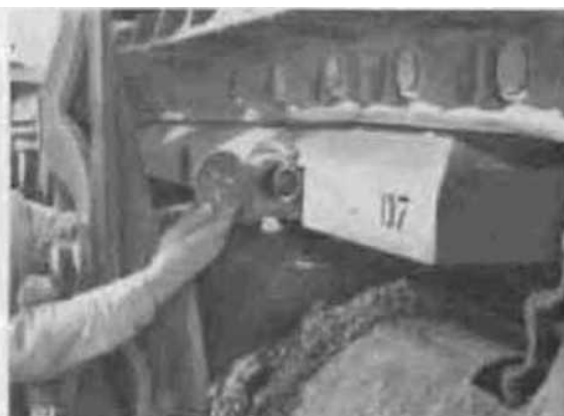
Figure 108. Installation of track support block.
