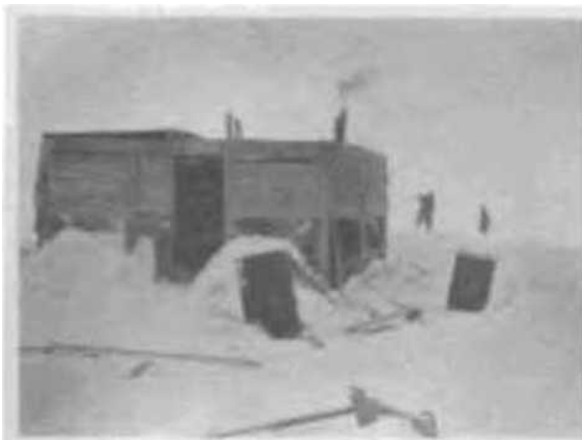
Figure 200. The snow melting plant.
