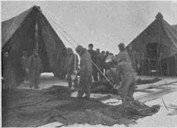
Figure 32. Erecting mess hall and kitchen tents.
