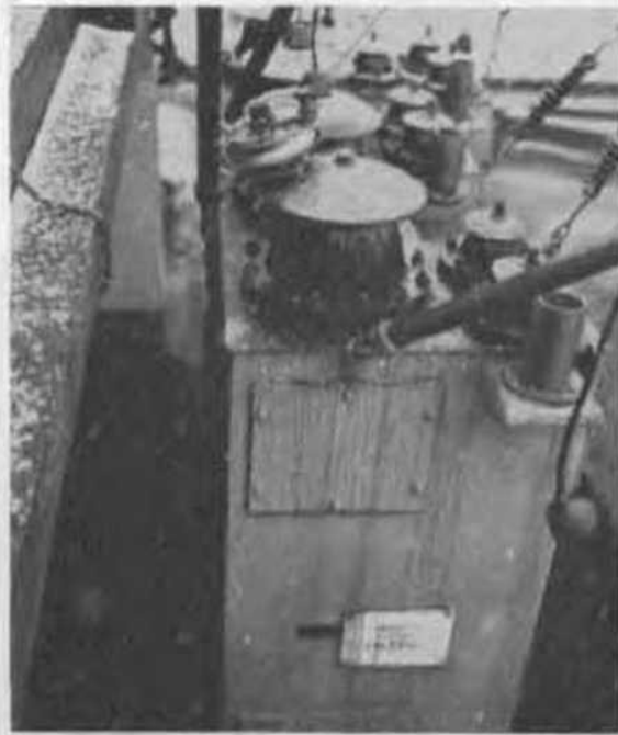
Figure 210. Antenna lead-ins on Mount Olympus.
