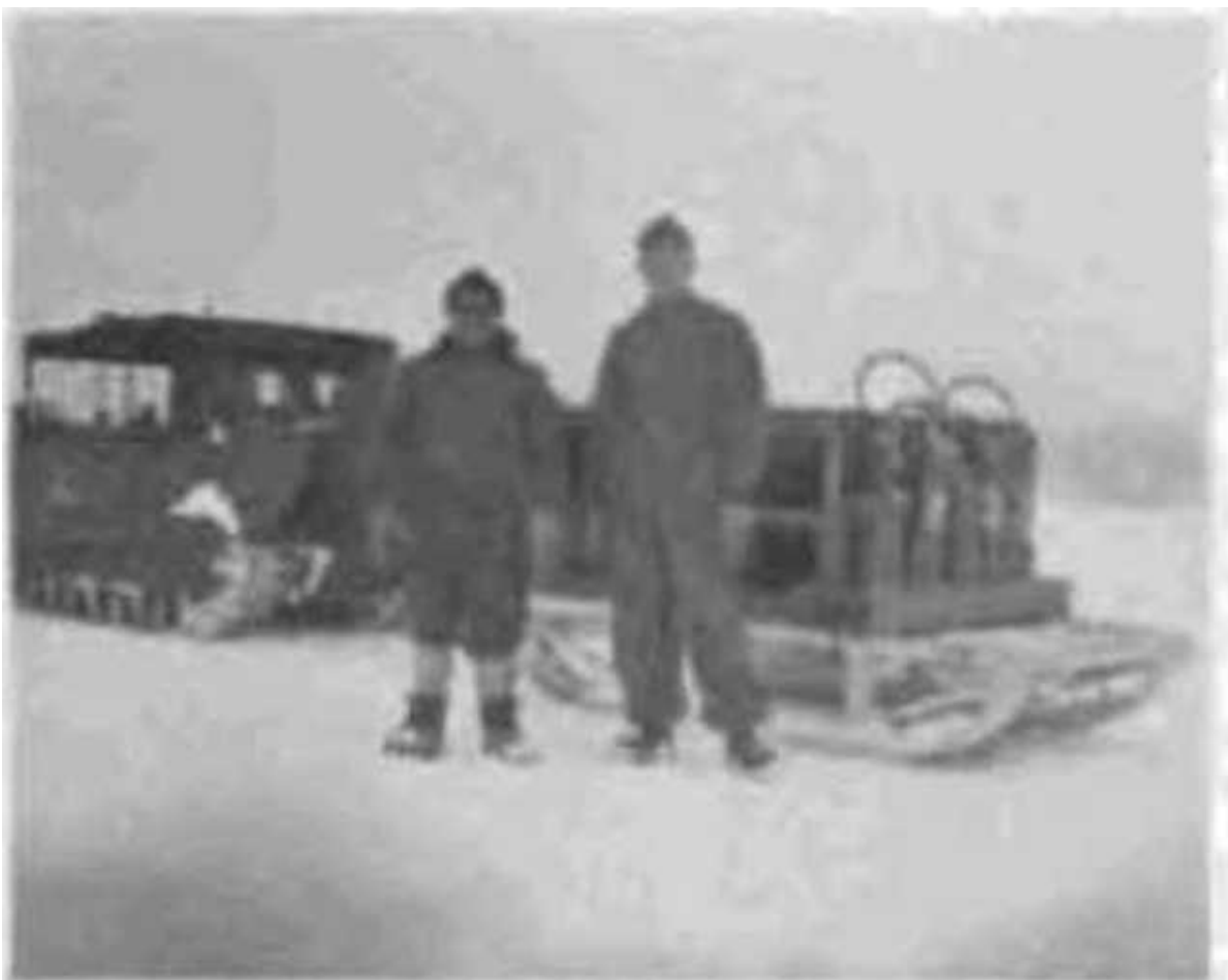
Figure 94. Weasel and 1-ton Army sled used at airfield as combination ambulance and crash truck. Note fire extinguishers.
