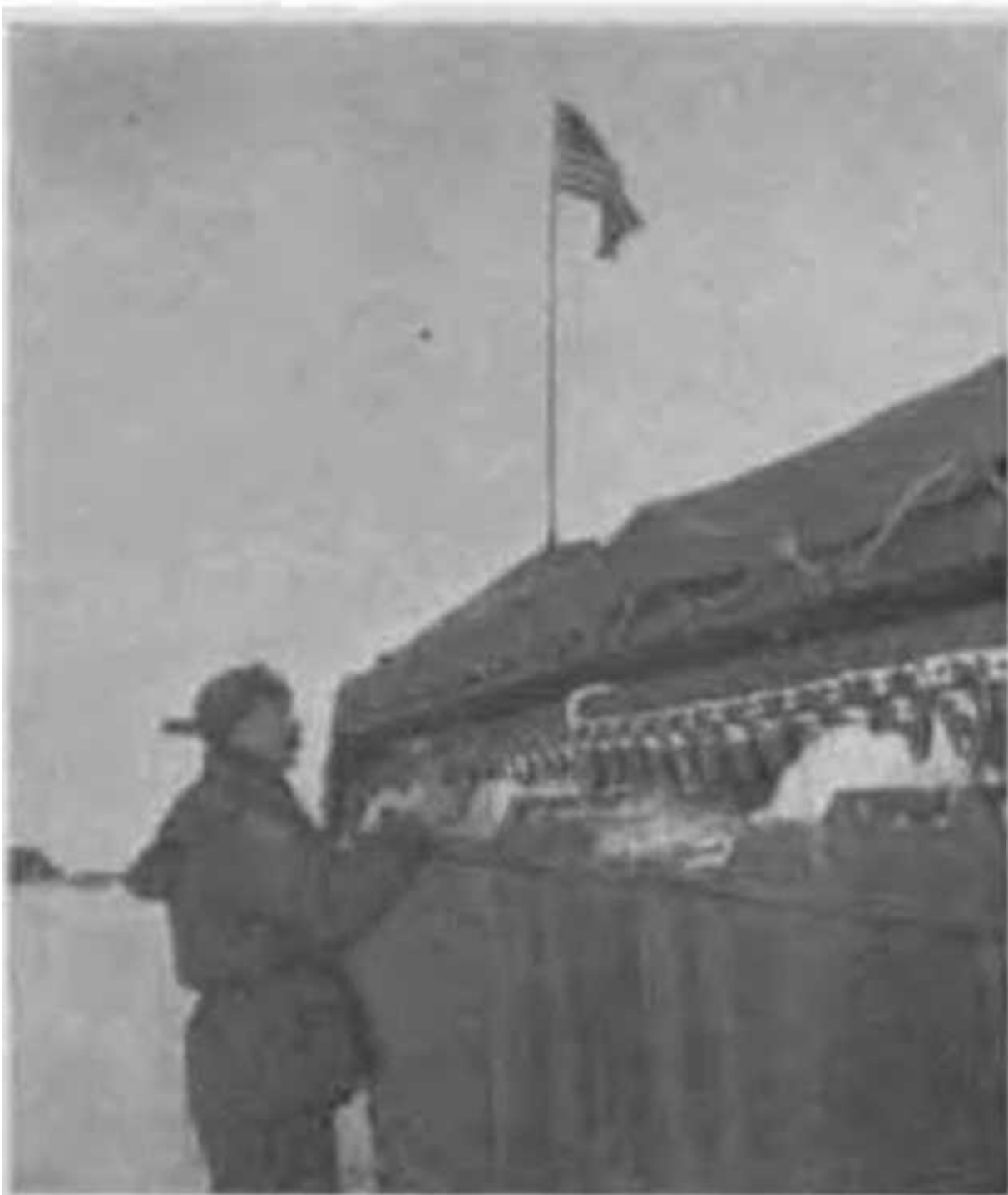
Figure 134. Keeping track and rollers free of ice and snow is important in the Antarctic.
