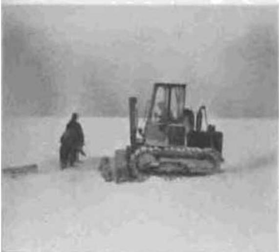
Figure 97. Fingerlift digging out pierced plank buried in snow.
