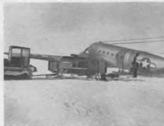
Figure 25. Aviation gasoline tank on skis was used to refuel R4D's (D-47's).
