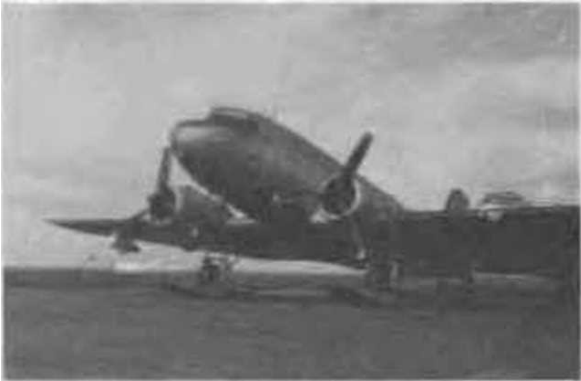
Figure 158. Navy R4D (Army C-47) type aircraft on flight deck of U. S. S. Philippine Sea (aircraft carrier) prior to take-off from ship to Little America. Note ski-wheel combination, necessary for take-off from flight deck and landing on snow surface at Little America.
