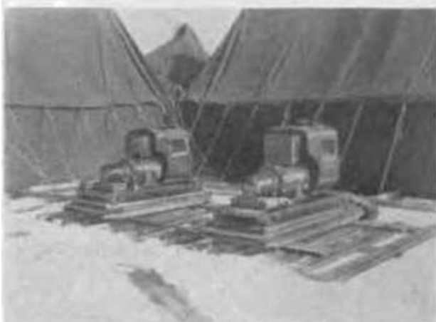
Figure 225. Camp lighting supply.
