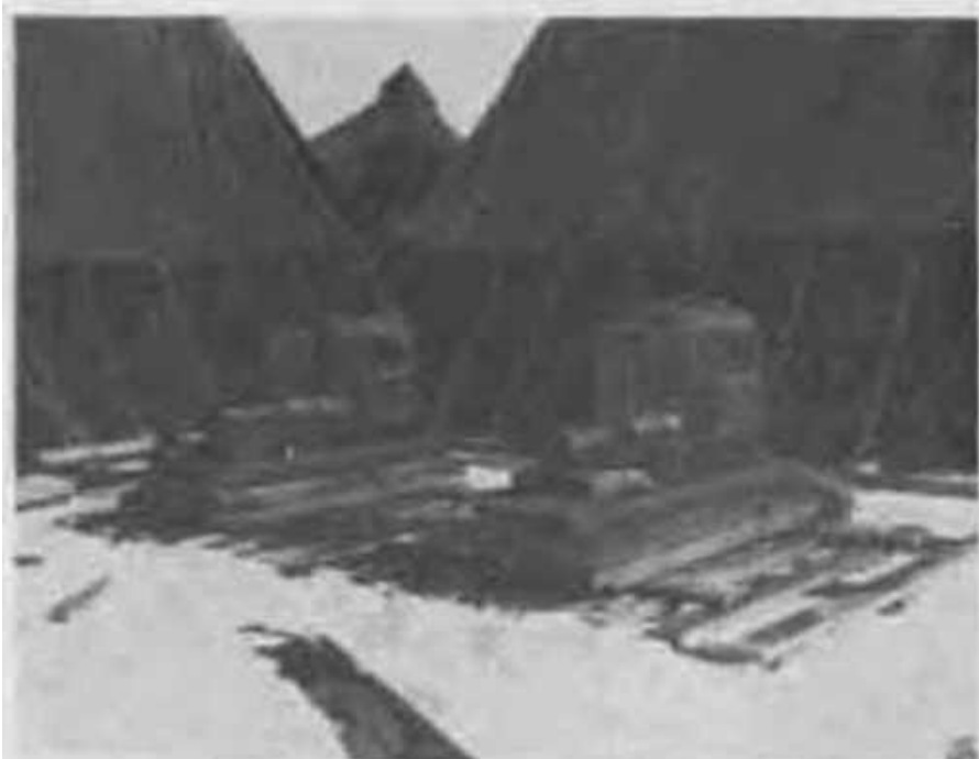
Figure 50. Two 5-kw. generators which were used for lighting kitchen and mess hall. Note they are resting on the base for a tarpaulin which was later erected.
