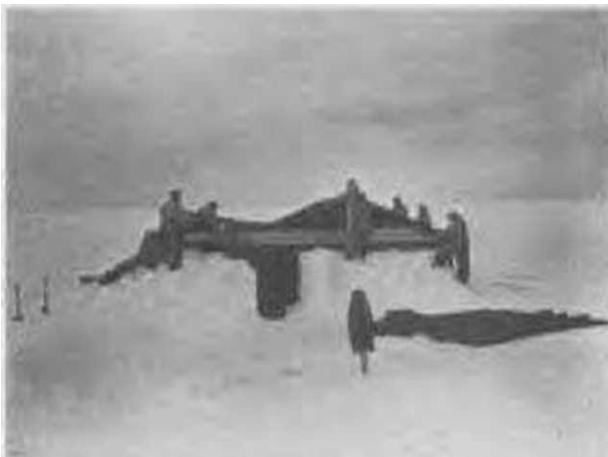
Figure 173. Construction of cold food storage room.
