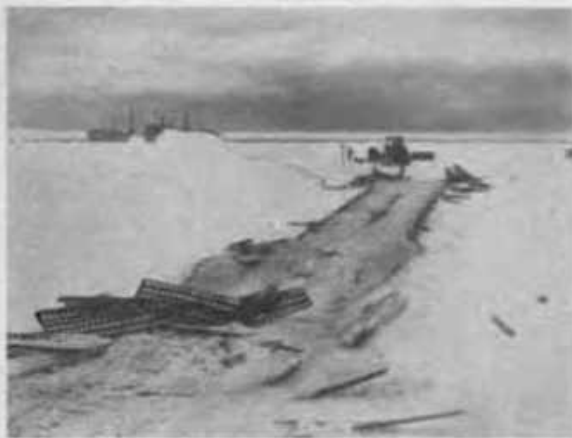
Figure 21. Damaged PSP on bridge which crossed crack in bay ice was later removed.
