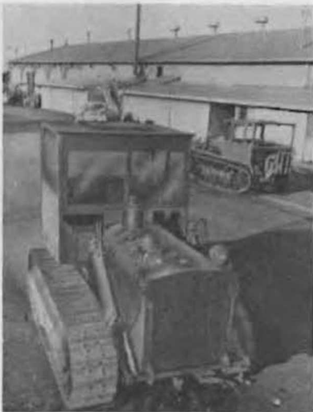
Figure 6. Winterized D-6 caterpillar tractor.
