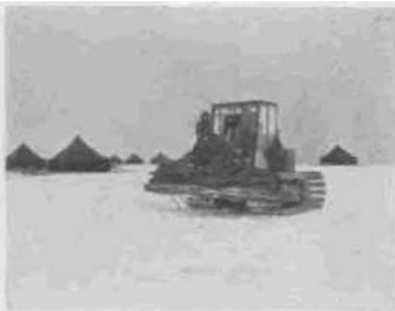
Figure 96. Load of lumber and tarpaulins on fingerlift.
