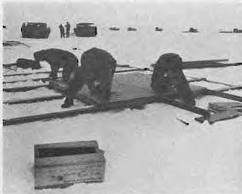
Figure 31. Assembling pyramidal tent floors. Note piles in background. Each is the required material for one pyramidal tent.
