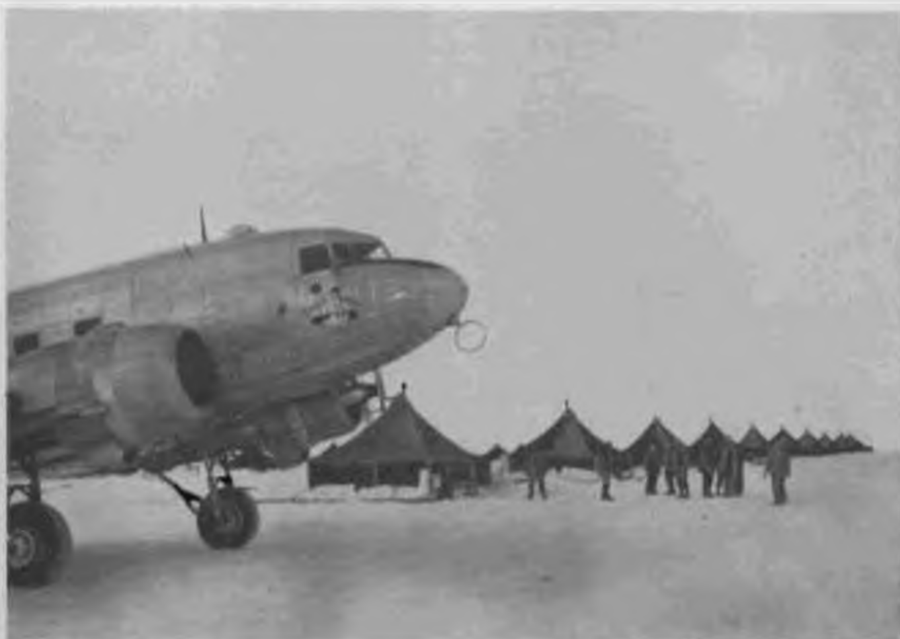
Figure 67. R4D (C-47) taxiing on main camp road leading to mess hall. No failure whatsoever was noted in surface.
