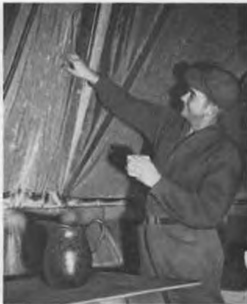
Figure 196. Interior view of mess tent, showing accumulation of frost.
