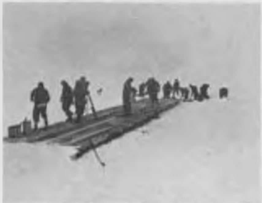
Figure 19. Bridge crossing crack in bay ice (PSP was put on top of one of the two bridges as wearing surface).
