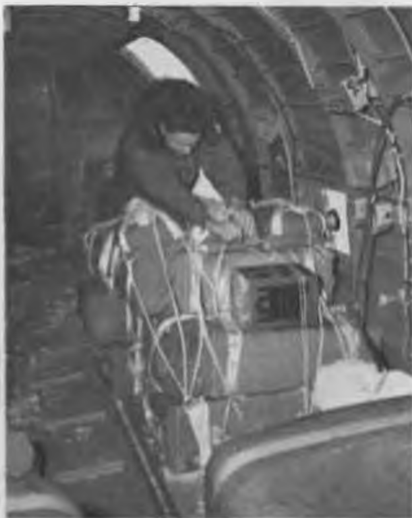
Figure 159. Emergency rations and equipment being lashed down in C-47 prior to flight. Note corner of Tokyo tanks in foreground.
