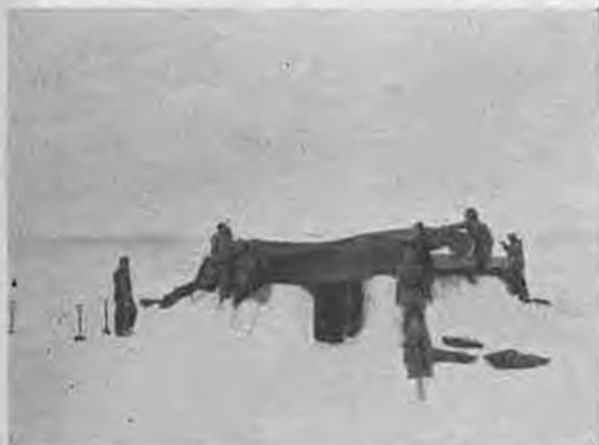
Figure 40. Tarpaulin being pulled over framework of frozen food storage house. It was weighted down by putting dunnage and snow blocks on top.
