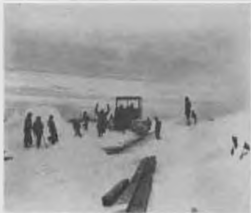
Figure 18. Tamping snow on a bridge with a tractor.
