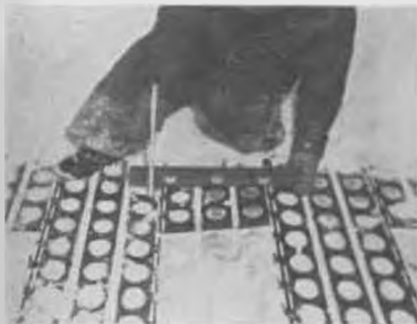
Figure 53. Same junction as in figure 52, showing that difference in elevation at this point is 2\frac{1}{2} inches.
