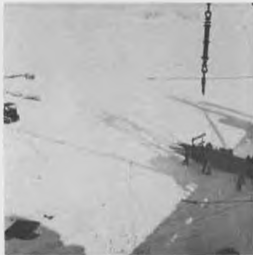
Figure 17. Unloading lumber from ship directly onto "Go-devil" sled (lumber to be used to construct bridge across cracks in bay ice). Note tractor staying away from ship's side in order to prevent danger of cracking edges of ice.
