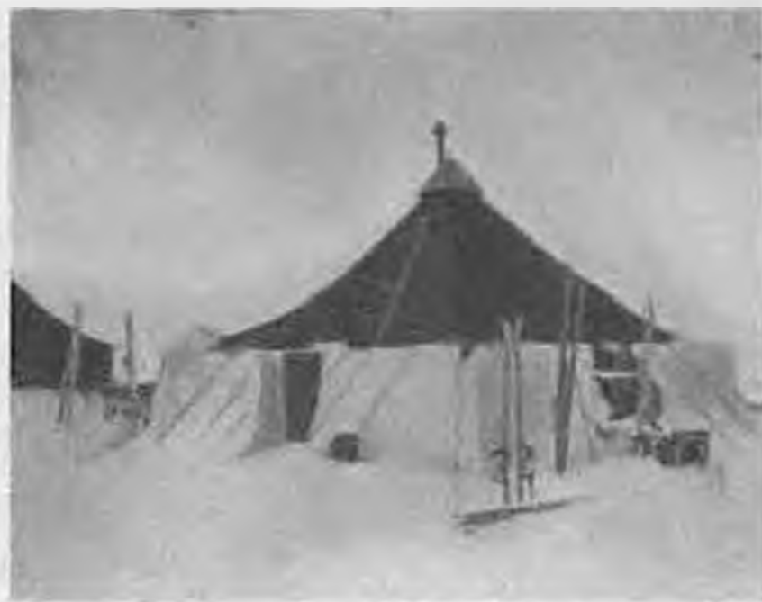
Figure 183. Living quarters, showing wall of snow blocks around entire tent for insulation purposes.
