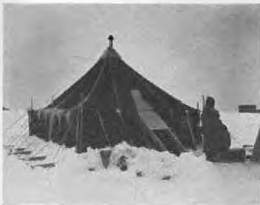
Figure 182. Living quarters, showing base frame of two-by-four's.
