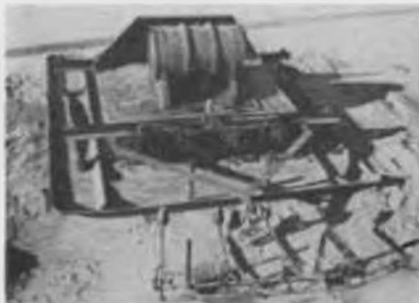
Figure 15. Snow surface heater with extra burners.
