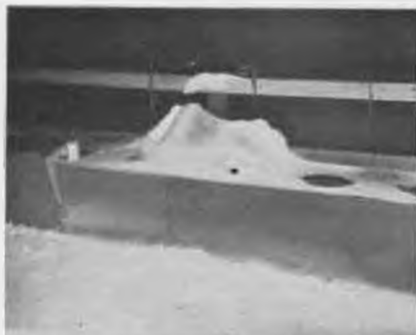
Figure 172. Interior view of latrine. This drifting occurred only during strong winds.
