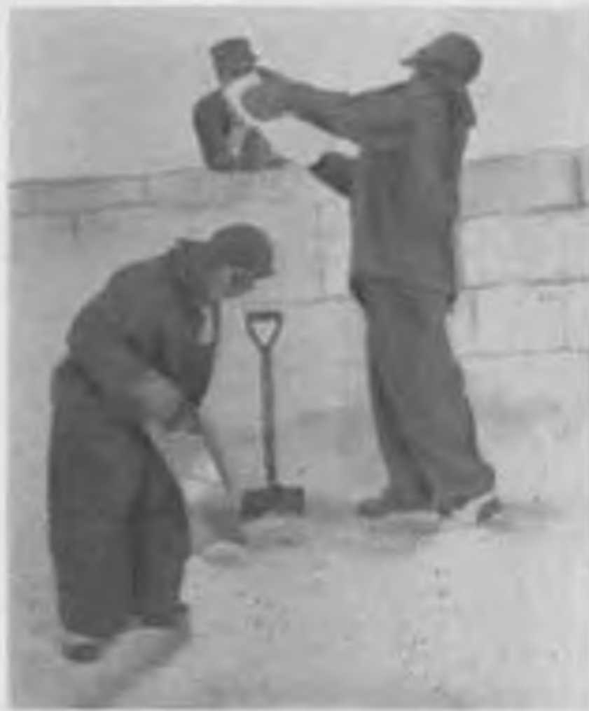
Figure 37. Digging hole for frozen food storage. Note snow being sawed into blocks for easier handling.
