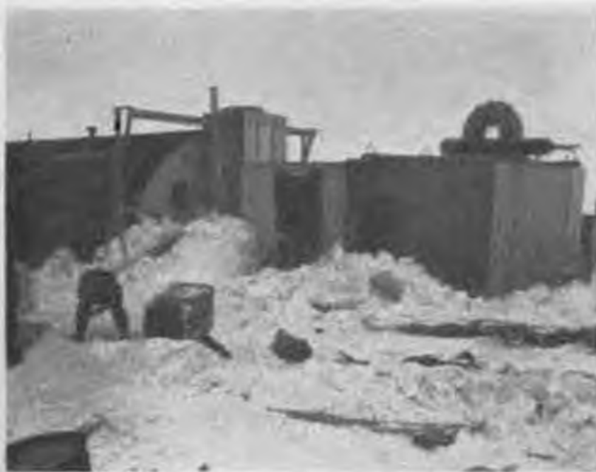
Figure 45. Southwest end of double Quonset hut at Little America III (35-man winter camp) showing escape hatch, short connecting tunnel, and generator house on right end.
