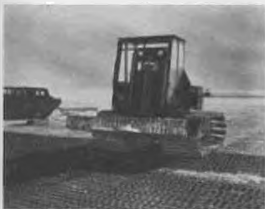
Figure 95. Fingerlift distributing pierced plank on the airfield.
