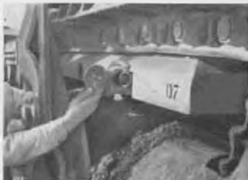
Figure 108. Installation of track support block.
