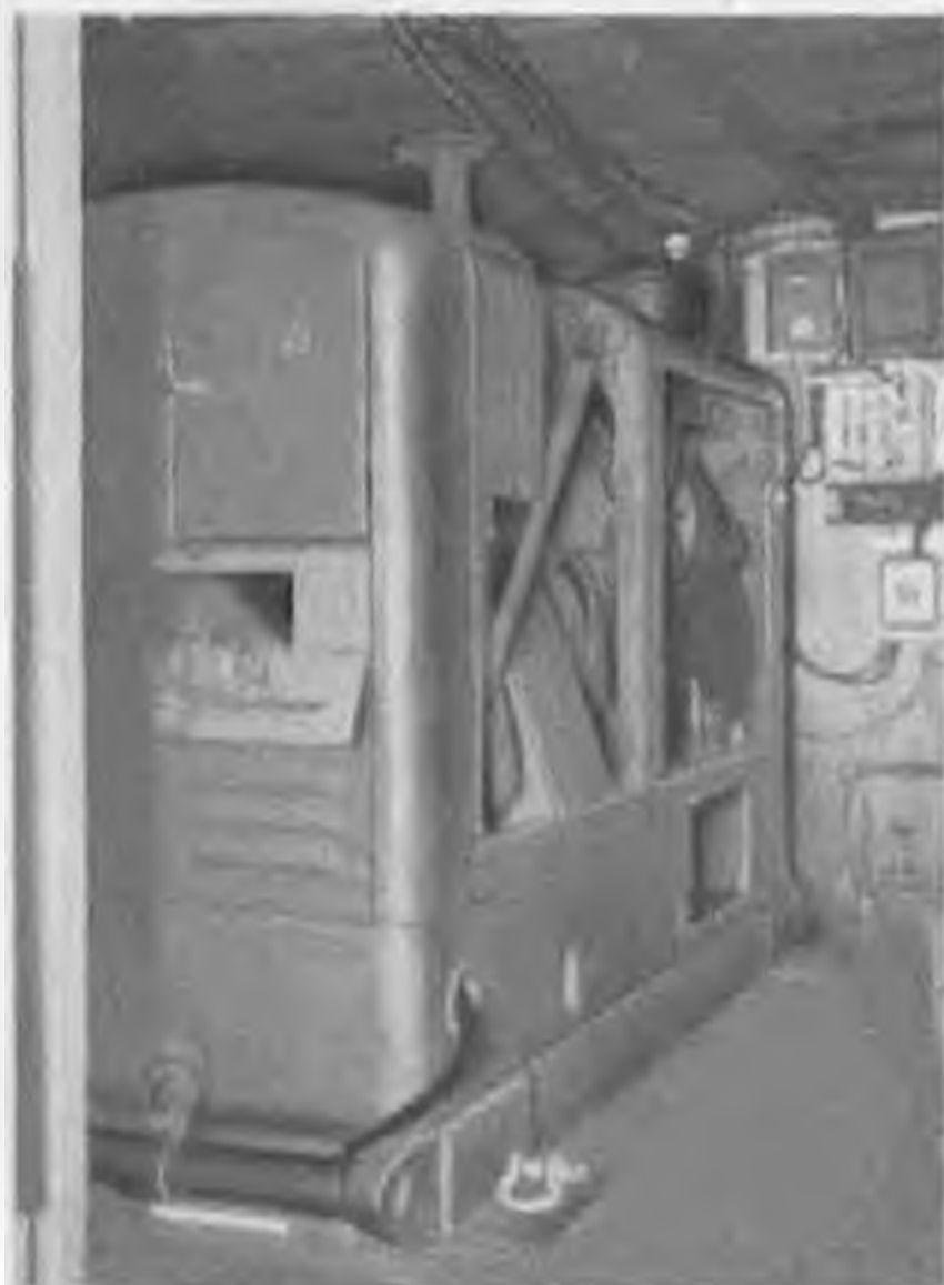
Figure 236. GM 25-kva. power unit.
