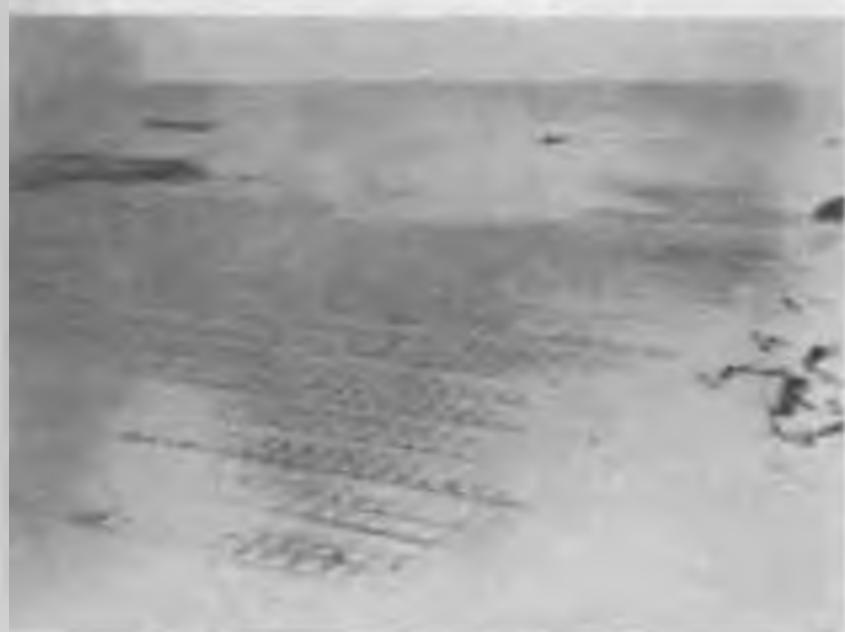
Figure 55. PSP test strip after a blizzard. Note drifts which were caused by bundles and odd pieces of mat left within area. This shows the runway areas must be policed as work progresses.
