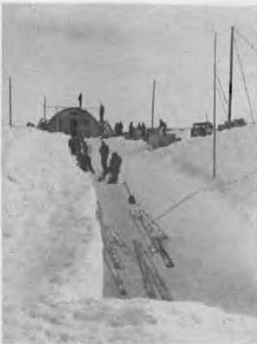
Figure 44. Looking southwest. Excavation for connecting tunnel leading from double Quonset hut in background to Little America III, which is beneath the photographer who took the picture.
