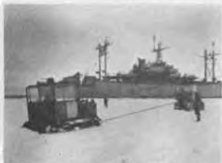
Figure 104. D-6 in trouble on bay ice about to be winched out by another D-6.
