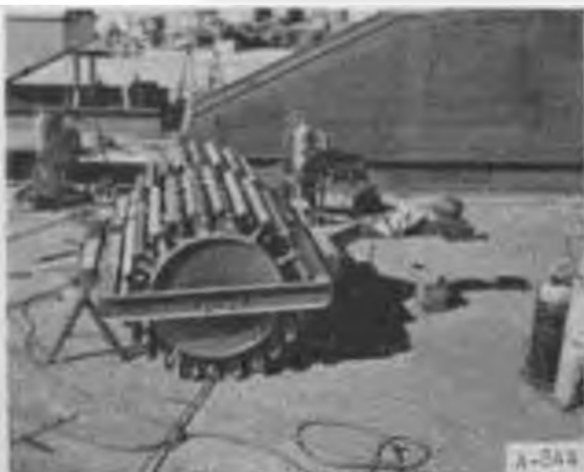
Figure 83. Modified sheepfoot roller (not used).
