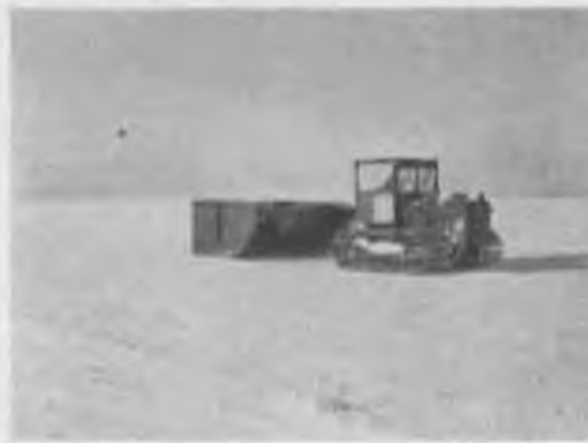
Figure 56. Tractor pulling pontoon drag on ski runway.
