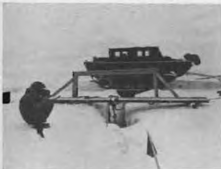
Figure 22. Footbridge and weasel bridge crossing crevasse which developed two-thirds of the way up barrier slope.
