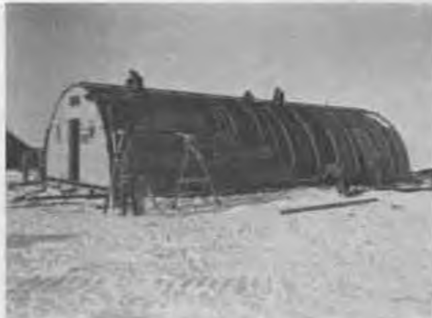
Figure 43. Quonset hut at base operations under construction. Note inside wall of Quonset hut at far end, outside corrugated sheets on left end and insulation which goes between the two surfaces being applied in the middle of the building.
